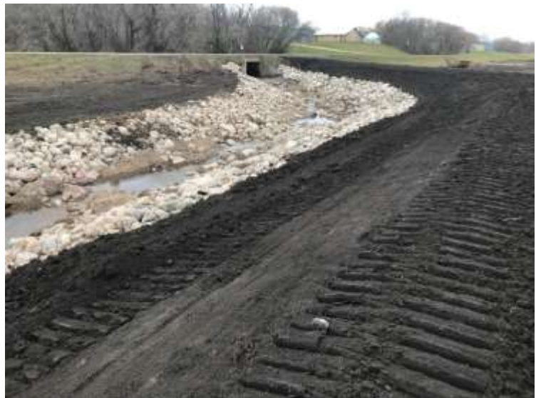
Phase 2 Looking East
