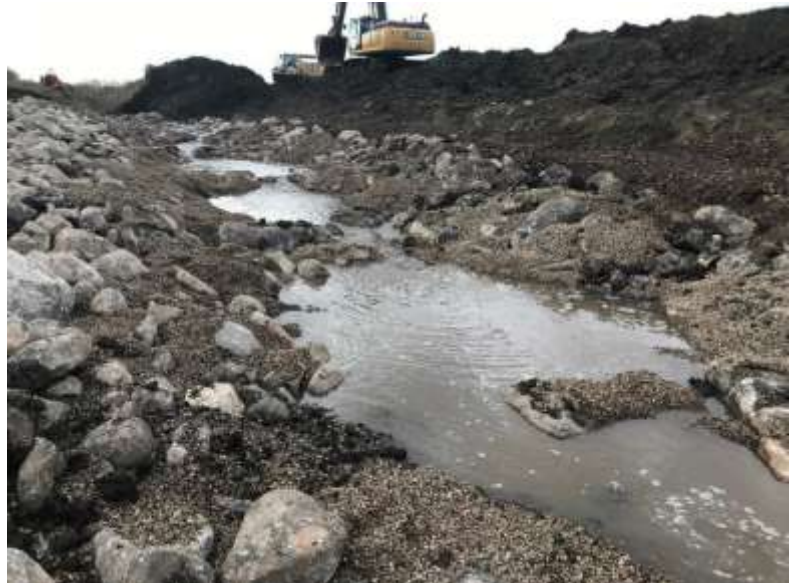
Phase 2 Rock Riffle Installation
